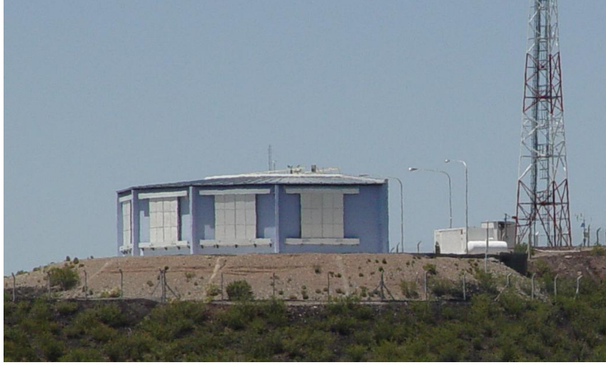
Figure 3.3: One of the four fluorescence telescope buildings.
